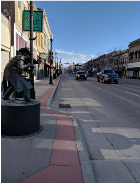
Existing curb extensions on Main Street in Sheridan are narrow in width.
