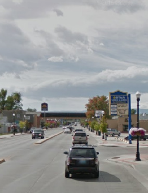
North of 1st Street, the cross-section of Main Street will remain as-is, as this section of roadway was reconstructed by WYDOT in 2011.
