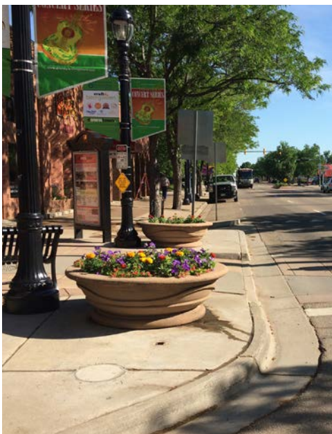
Wider curb extensions that extend the full width of the on-street parking lane in Longmont, Colorado, offer space for a wide variety of street furnishings and shorten the crossing distance.
