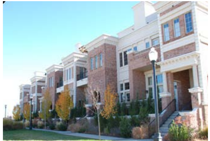
Image 25. Touchstone Homes in Stapleton in Denver feature urban brownstones, which bring New York City to suburban Colorado. Photo by Touchstone Homes.
