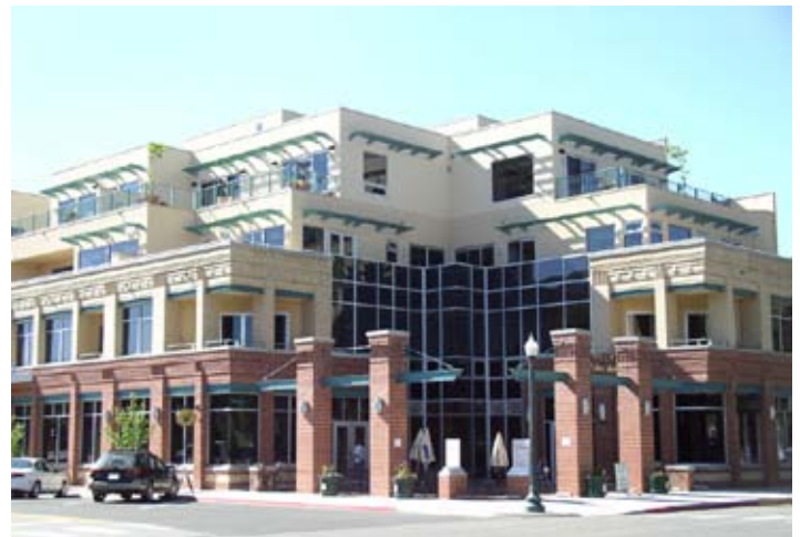
Image 21. 1201 Main in Durango, Colorado is home to 22 lofts and five commercial/office units. The property is popular among many different age groups, empty nesters are driving the success of the development. Photo by Feeney Architects.
