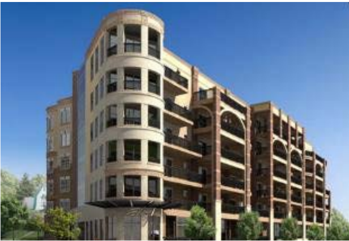
Image 22. RiverClay Condominiums represent the Rocky Mountain region's first LEED-certified multi-family project, located in Jefferson Park, Denver, Colorado. It includes 60 residential units with two commercial units in a six-story building totaling 138,000 square feet. Built by Zocalo Community Development.
