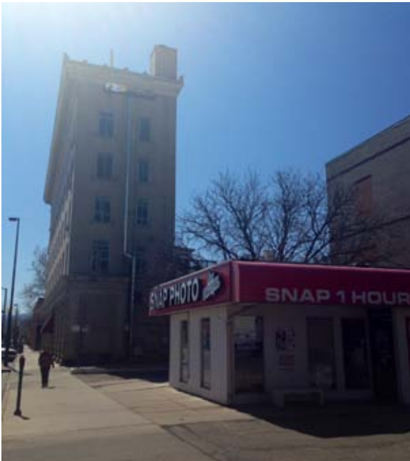
Image 14. Existing building located in the east Rood Avenue endcap.
