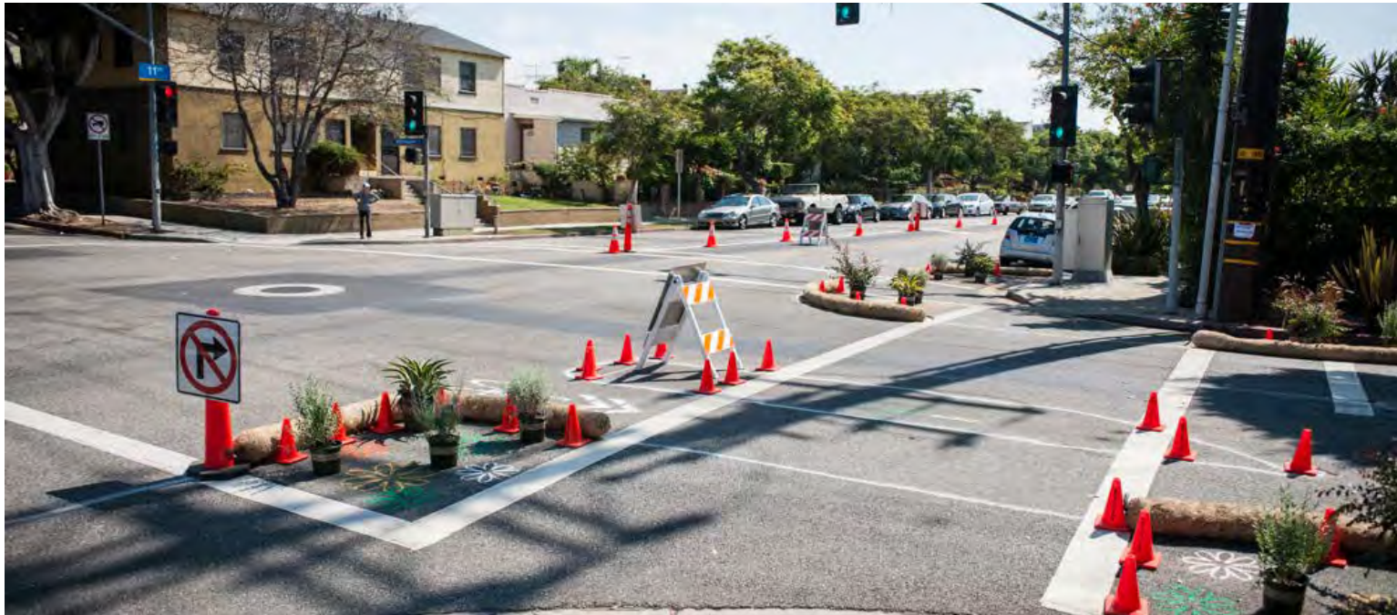
LQC techniques should be used to test Main Street intersection treatments before made permanent adoption
