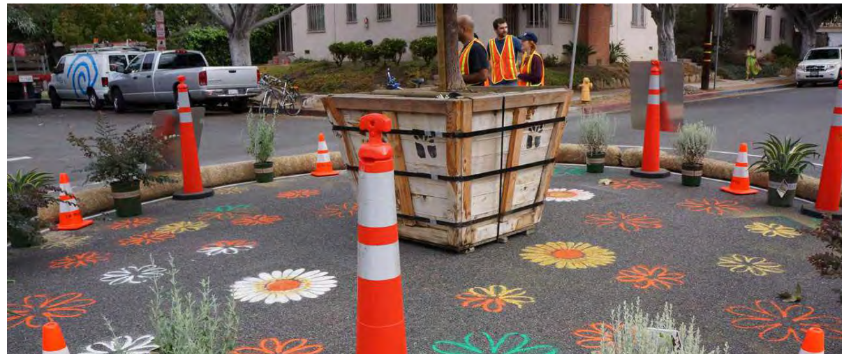
LQC roundabout treatment using straw wattle, traffic cones, chalk, and tree
