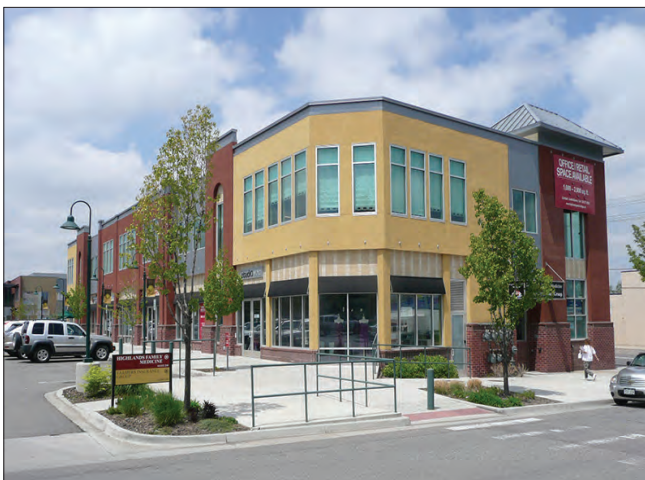
parking at the side or rear of buildings is desired as illustrated in the Denver example
